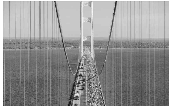
For the first time in its 60-year history, one of the Mackinac Bridge's iconic ivory towers will be stripped down to bare metal and repainted. MDOT PHOTO
